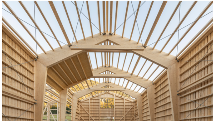
Fig. 4: Engineered wood that has parallel wood laminated glued together. Often used in combination with CLT when more flexibility is needed and when there are big open spaces (e.g. offices)
